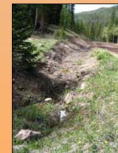
Drainage embankment from road
